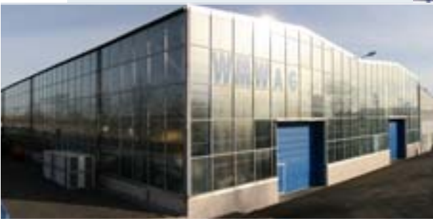
The glazed exhibition halls of the used-machine dealer WMW AG in Leipzig are full of life pictures: WMW
